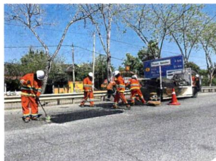
For the period between Sept 1 and Nov 30, as much as 15,973 or 100% of the potholes on federal roads spanning East and West Malaysia were patched within 24 hours.
